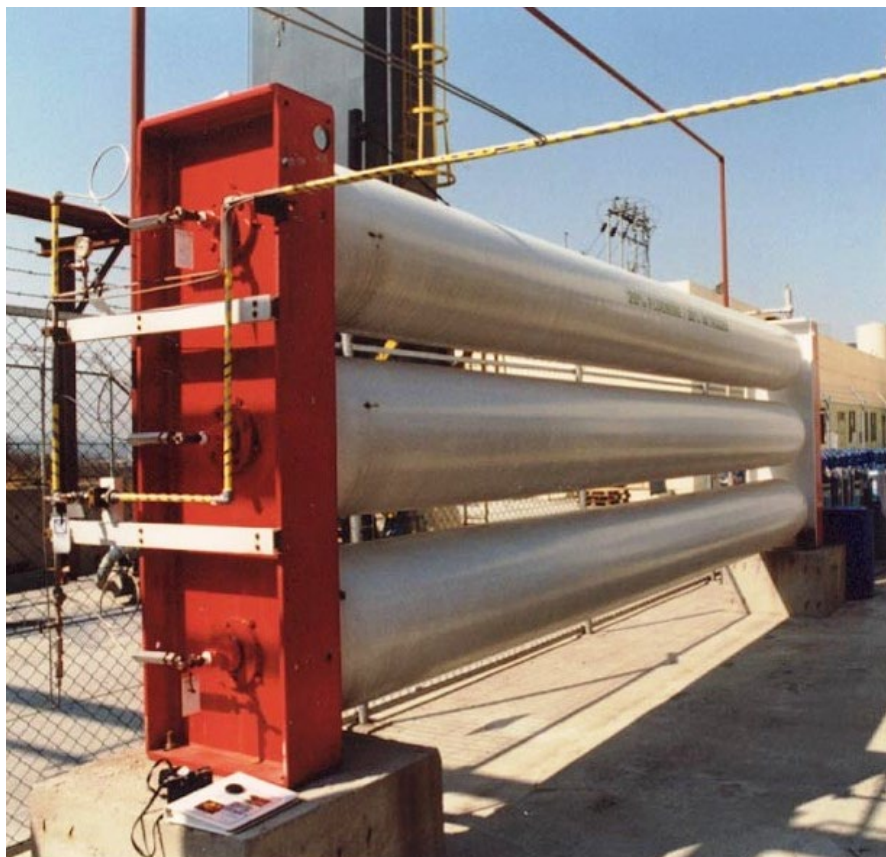
Figure 2: Typical Ground Tube Installation
